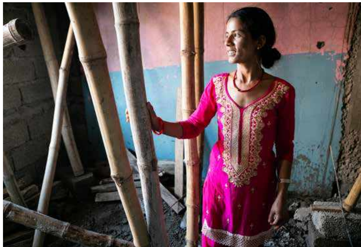
Raj Kumari and her husband took out a loan with WSDO to be able to build their first house. She proudly shows how construction is going and says that it will be ready in five months for the whole family to live in.
